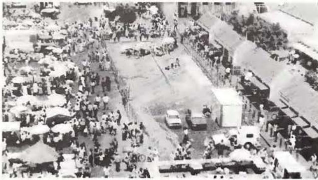
Fig. 2. The position of excavations next to the existing stalls on the Grand Parade, 1991. Photographed from the roof of the Golden Acre. (Photograph by G. Abrahams-Willis).
